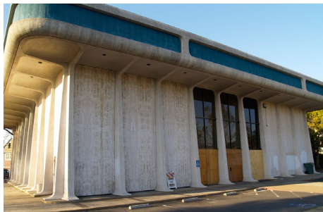
Battered by vandals and a shifting economy, the Global Video building now stands empty. PHOTO: RNEWS
