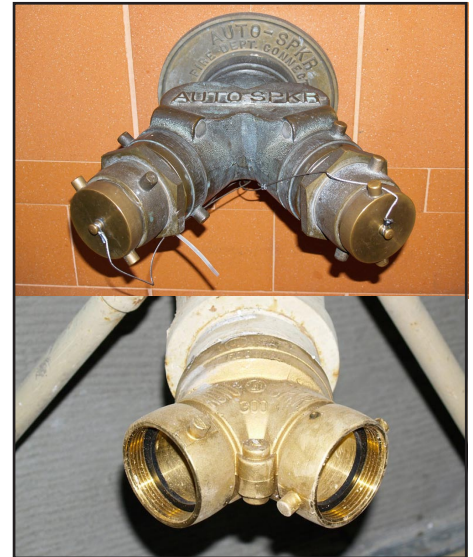
Siamese connectors, one with brass caps (top), one without.
