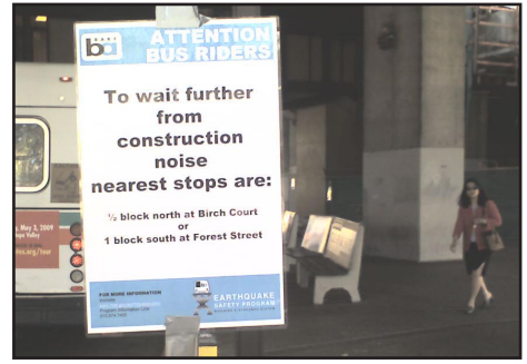
After RCPC identified dangerously high sound levels at BART’s construction site, the agency posted this sign.
