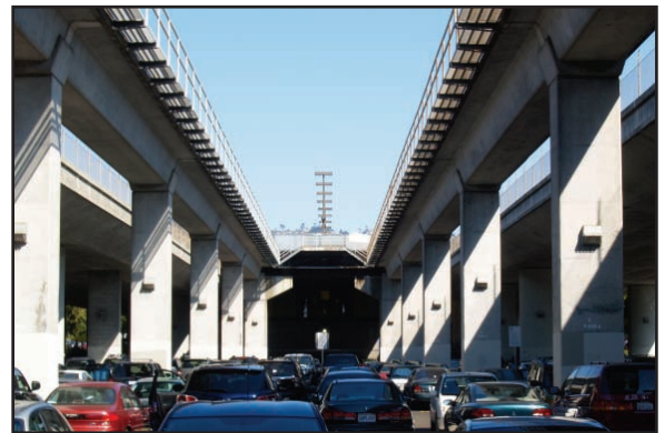
Come year’s end, BART will begin earthquake retrofit work on the Rockridge station and on columns supporting elevated trackways. Valet parking will be available to minimize disruption of commuter parking. PHOTO: DON KINKEAD
