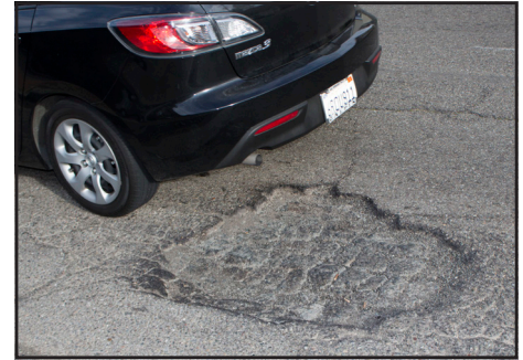
A driver escapes from the Claremont Avenue pothole near FROG Park measuring 3' wide x 4' long x 3" deep. /D. KINKEAD
