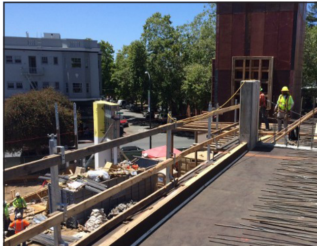
Safeway construction site above 63rd Street and College Avenue. /ELISABETH JEWEL
