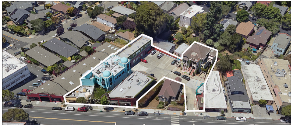
According to Jake Allen, son of the property owner, five buildings will be removed at 5295 College Avenue. Most of them have been rebuilt or redone within the last 50 years, and, as such, are structures of "little or no importance."
